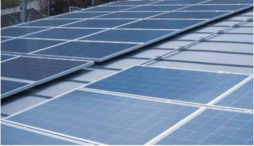
Elpo | Bruneck - Italy System: 66,24 kW | Seam metal with S5!
